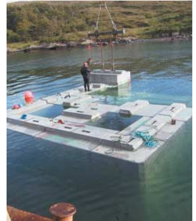
Small Isles Ferry Scheme. Photo courtesy of Construction Centre Group Limited
