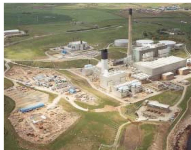
Peterhead Repowering Project. Photo courtesy of Siemens Power Generation
