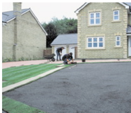
ScotAsh FBA is used as a surface for turf laying
