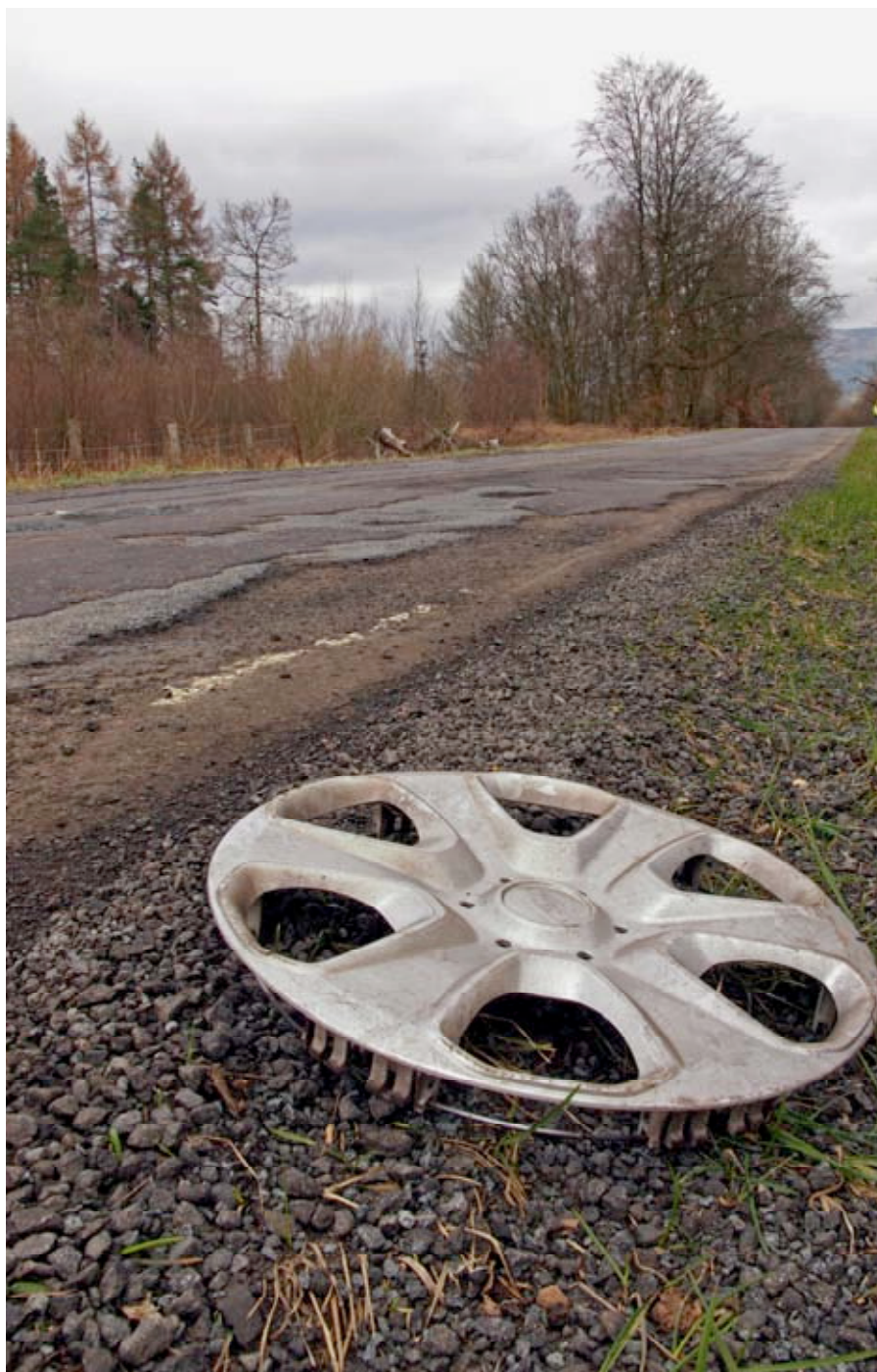
Erode to nowhere: The A81 main road had deteriorated due to frost damage, leaving it rutted and worn
