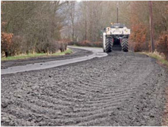
Road recycling in action: left, from top, the A81 is pulverised by Stabilised Pavement's Wirtgen 2000; ScotAsh's Hydraulic Binder is delivered in 30-tonne loads and transferred to the road recycler; the Hydraulic Binder next to a surface where the material has already been mixed with the recycled aggregate; and the road is levelled. Main pic, appropriate PPE is worn as the Hydraulic Binder is mixed in.
