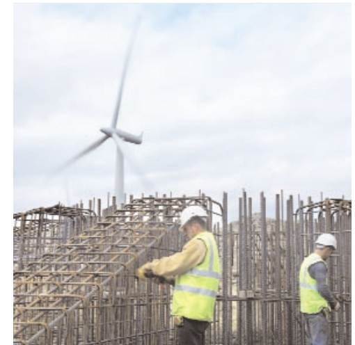
■ Preparing the base for a new turbine at Black Law
