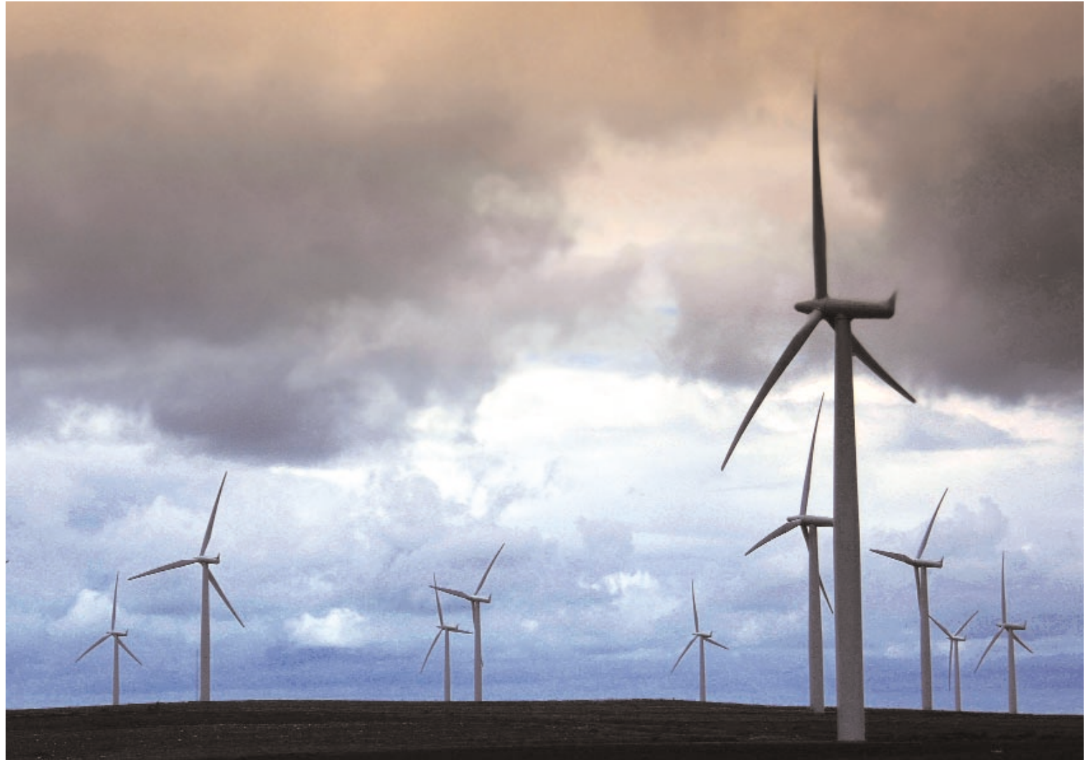
■ ScotAsh supplied cement products to Black Law windfarm in Lanarkshire, the largest operational onshore windfarm in the UK.
