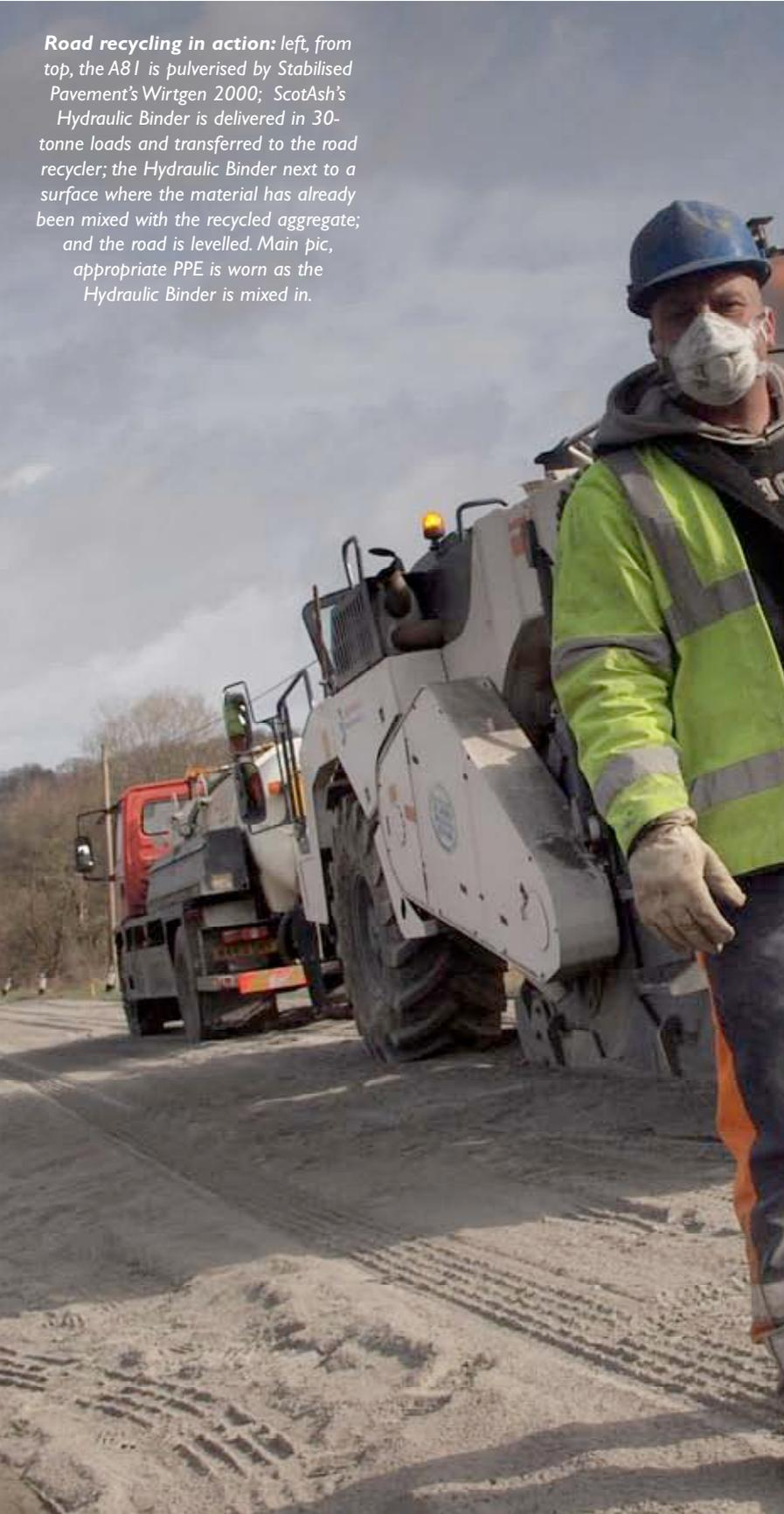
*Road recycling in action: left, from top, the A81 is pulverised by Stabilised Pavement's Wirtgen 2000; ScotAsh's Hydraulic Binder is delivered in 30-tonne loads and transferred to the road recycler; the Hydraulic Binder next to a surface where the material has already been mixed with the recycled aggregate; and the road is levelled. Main pic, appropriate PPE is worn as the Hydraulic Binder is mixed in.*
